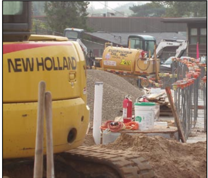
Top: Filling in the East Courtyard and getting ready to pour the big wall. The orange things are the ends of reinforcing rods that make the wall stronger. Below: Looking east at the new wall from the Findorff plan shed.
